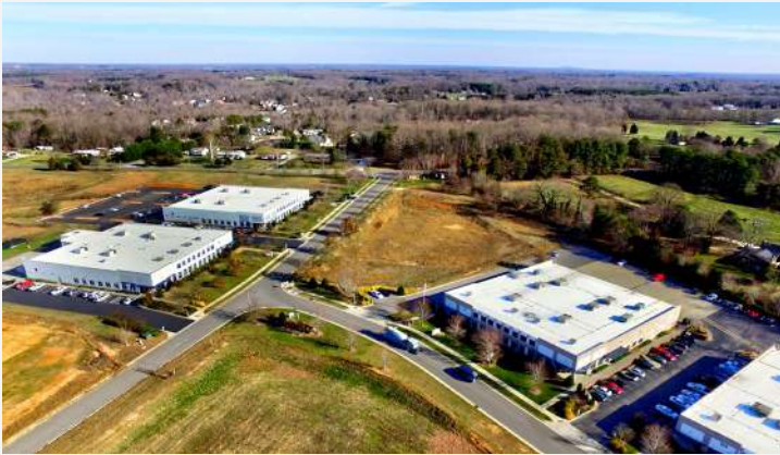
Main Entry at Cornelius Rd and Exmore Rd
